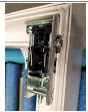
Screw the arm holder of the new support arm to the window sash fixing it with screws into the existing openings left after the previously disassembled holder of the old arm. (see item 7).
