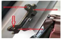
8 Drill the openings in the PVC profile for embossings in the holder according to the drilling template. Be careful, however, not to drill through the steel reinforcements.
